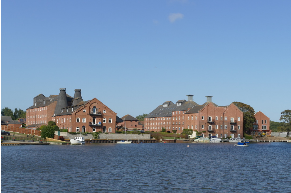
Converted warehouses at Oulton Broad
