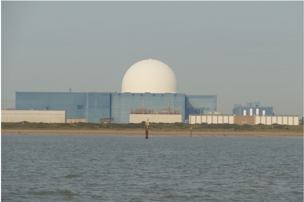
Sizewell B nuclear power station
