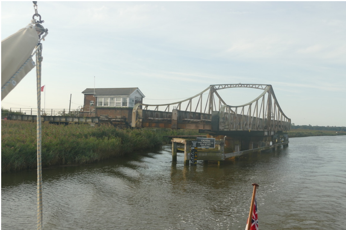
Somerleyton railway bridge
