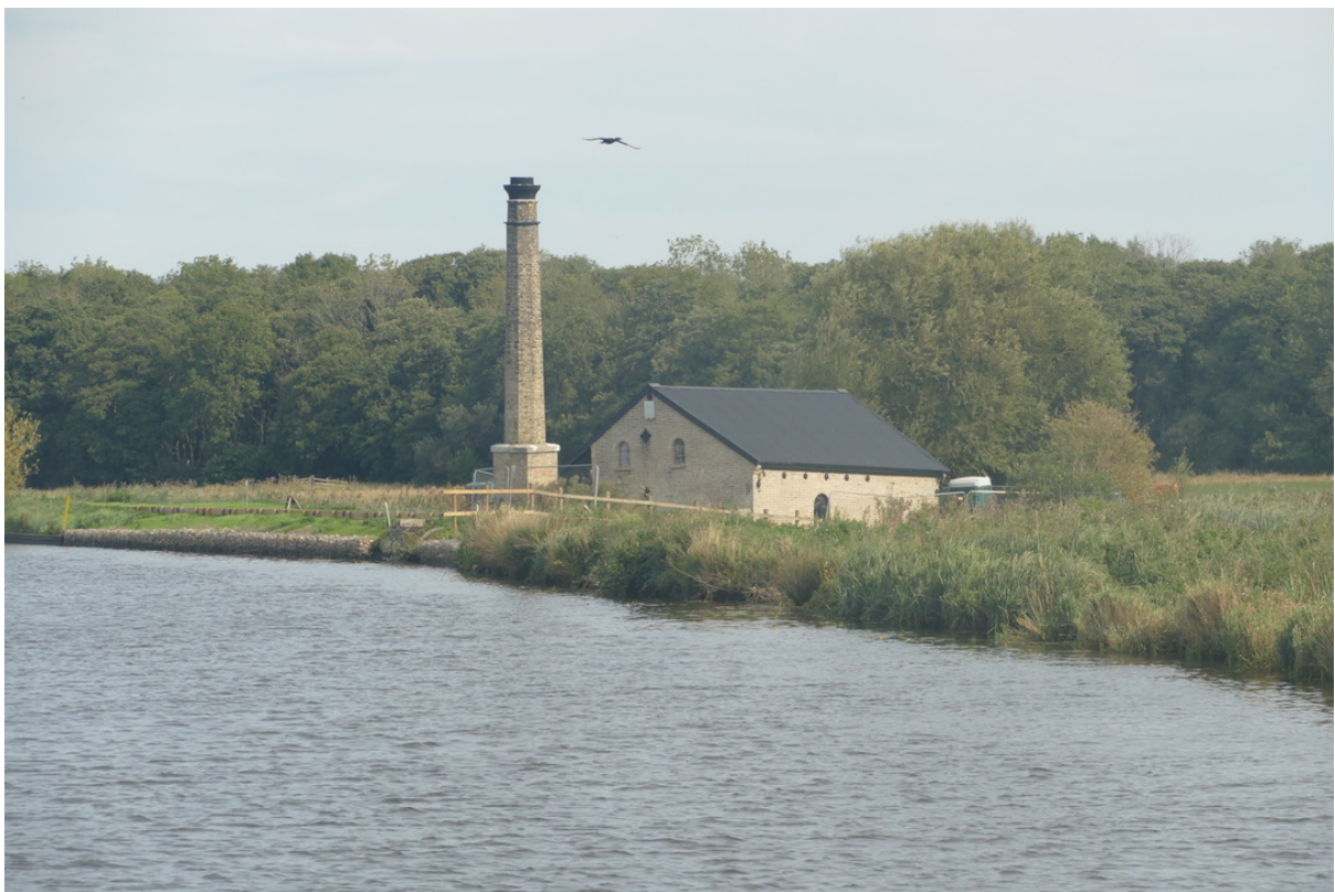
Former steam pump.
