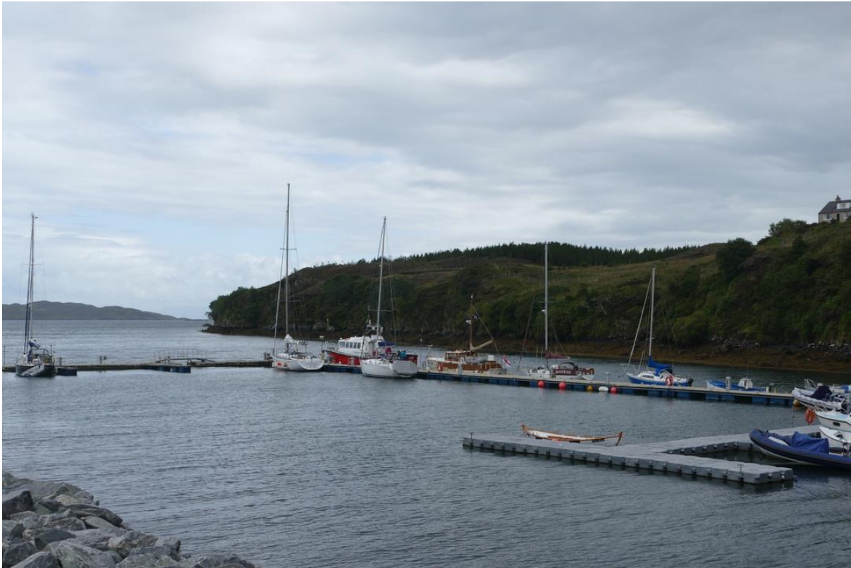
The pontoon at East Tarbert, Harris
